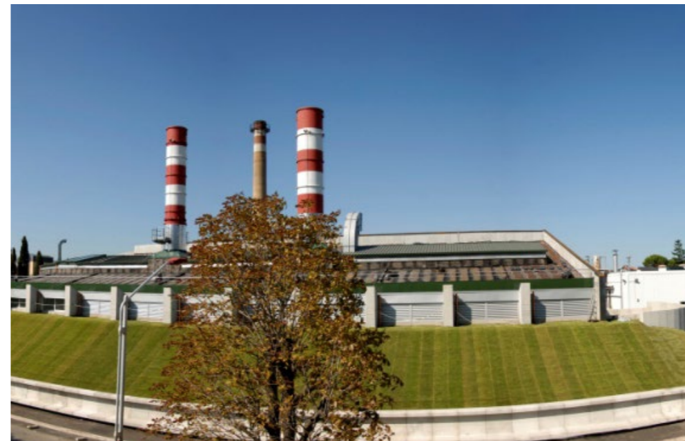
Trigeneration Plant of Careggi Hospital
